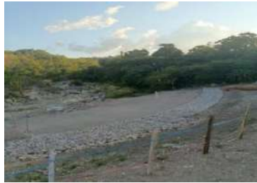
Figure 3. Gabions (mitigation facilities)
