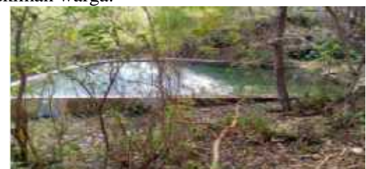
Gambar 3. Bak Broncaptering
