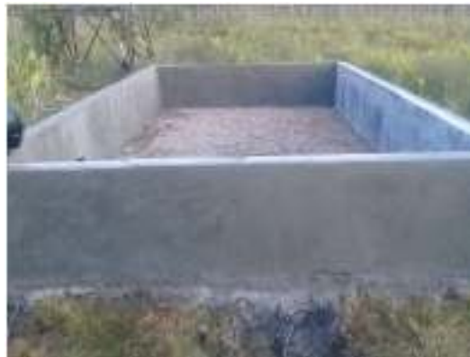
Figure 1. Ammonia and Silage storage tanks
