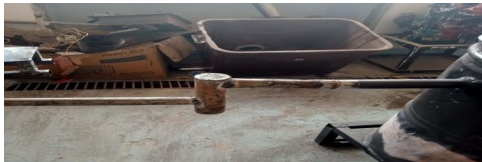
Gambar 3. Pipa distribusi gas
