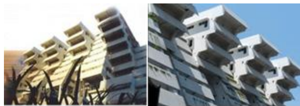
Gambar 7. Fasad Bangunan Intiland Tower Surabaya Sumber: https://www.archdaily.com/883921/unpacking-paul-rudolphs-overlooked-architectural-feats-in-southeast-asia (2017)
