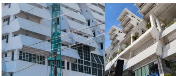
Gambar 20. Double Skin Façade Intiland Tower
