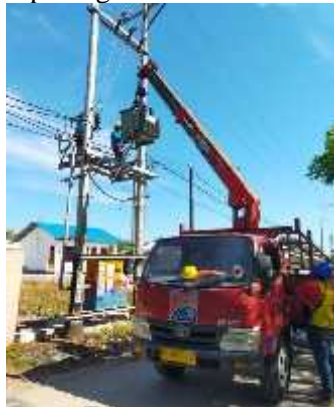
Gambar 2. Metode Uprating Transformator
